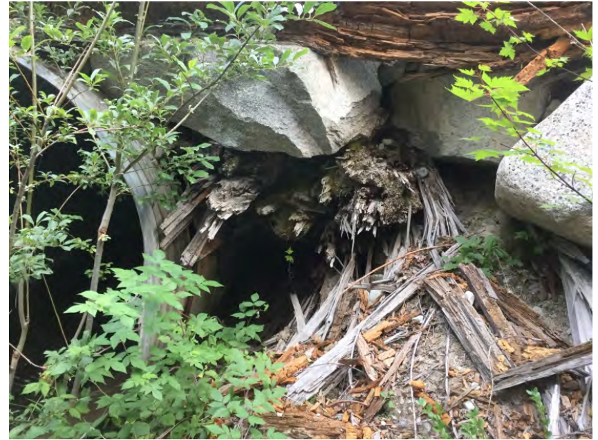
Logs were used as fill around culvert
