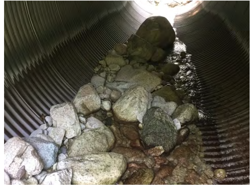
Material being transported into culvert
