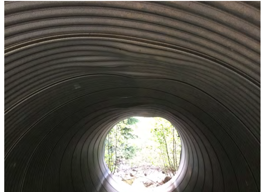
Minor roof damage
